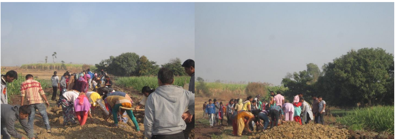
Road construction by NSS Volunteers
