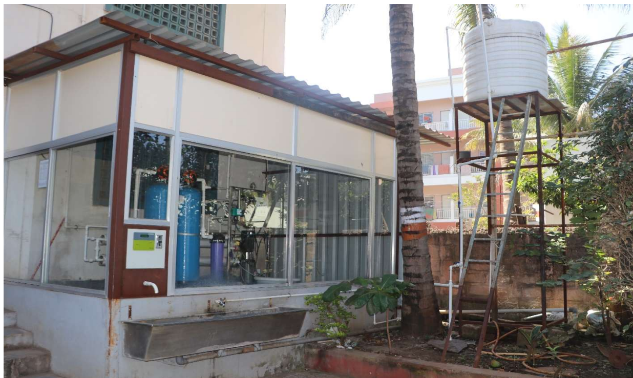
Drinking water facility
